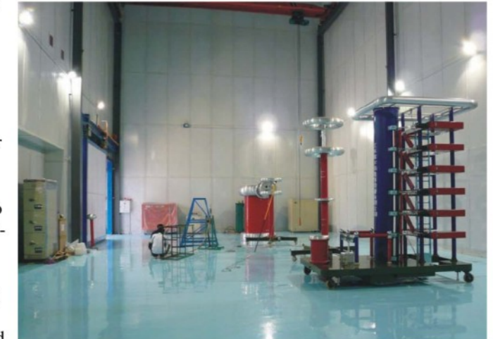
Tests in the high-voltage laboratory of WOER corporation
